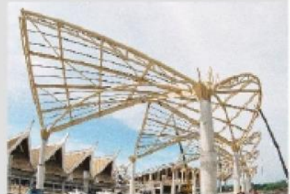
Steel Column Structures
