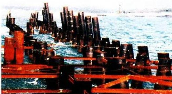
The pipe piles are normally manufactured from steel plates, which comply with Grade 43 or 50 of BS 4360, SS 41 or 50 of JIS G3101 or St. 44 or St. 52 of DIN 17100 with properties in accordance with the specifications as listed in Table 1.
